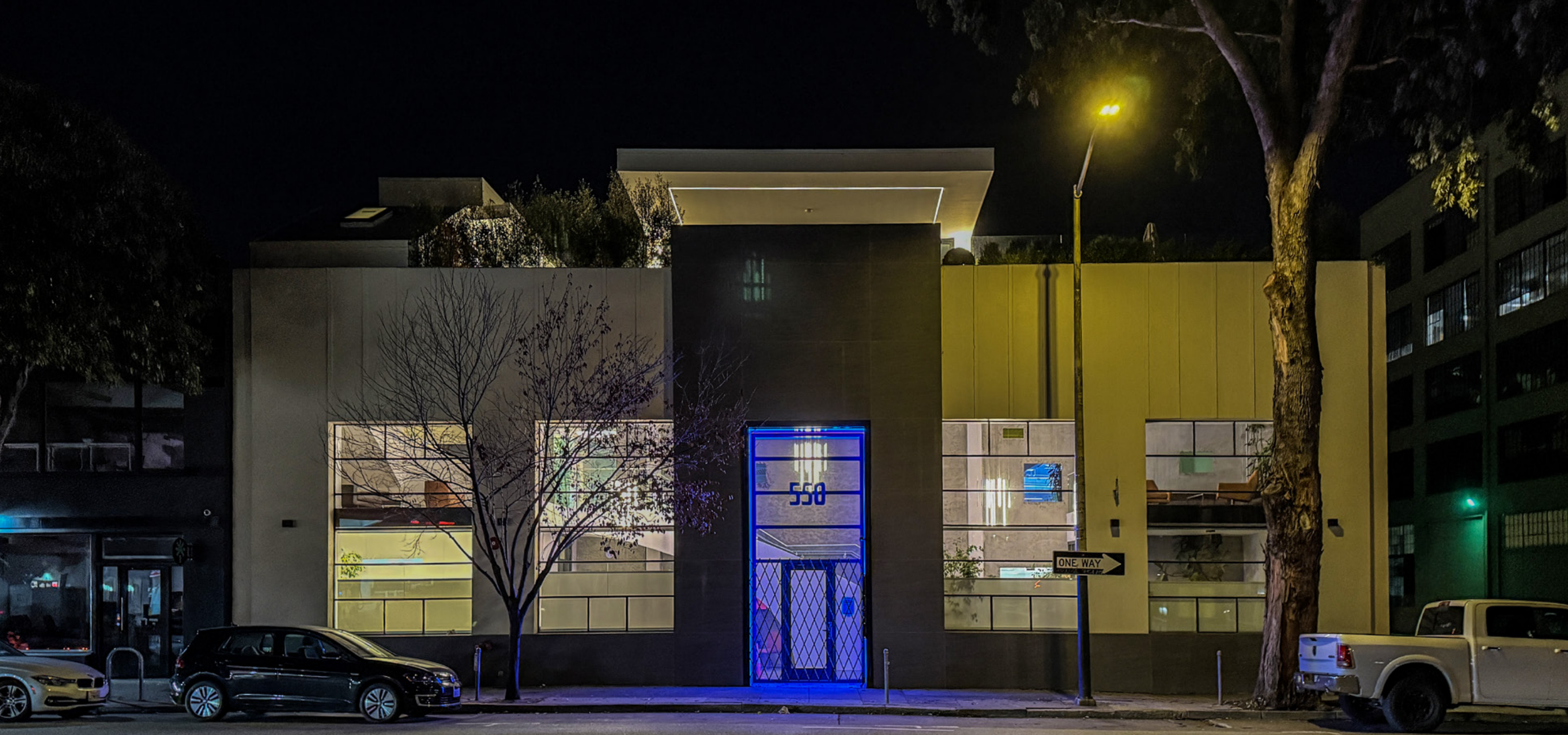
Front facade - New entry portal, stone cladding, penthouse, elevator & paint job (Built 2024)
